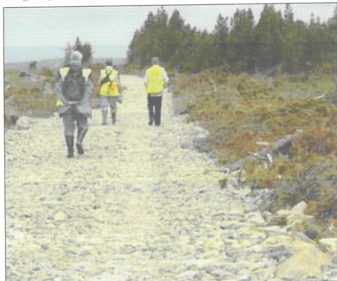
Plate 5.1: Floating road at Derrybrien Wind Farm.
